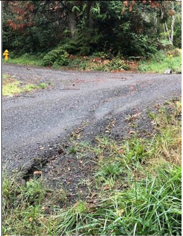
Phot shows road damage, ditch line failure, culvert failure at main road junctions with pump site access
