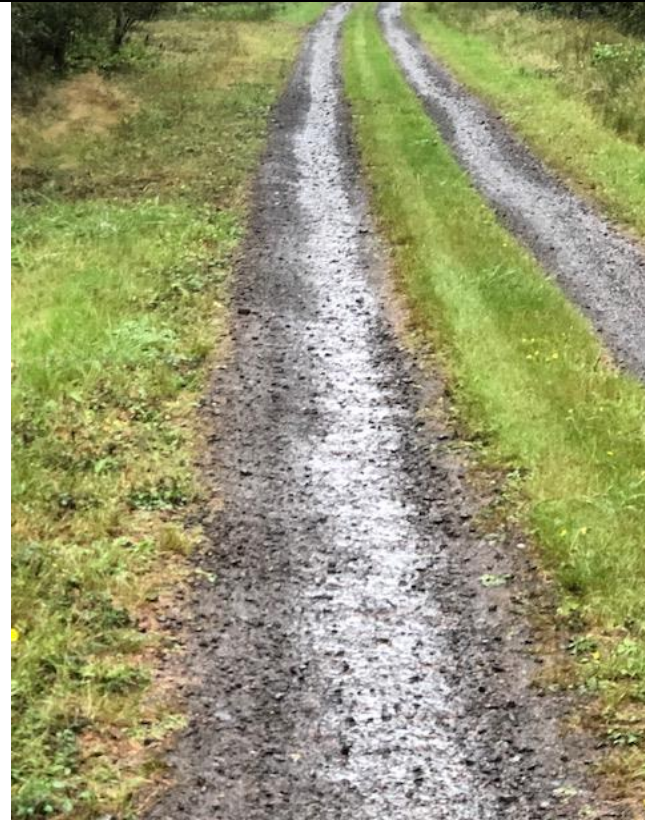
Photo top of hill looking east on access road shows channeling of storm water and worn wheel tracks
