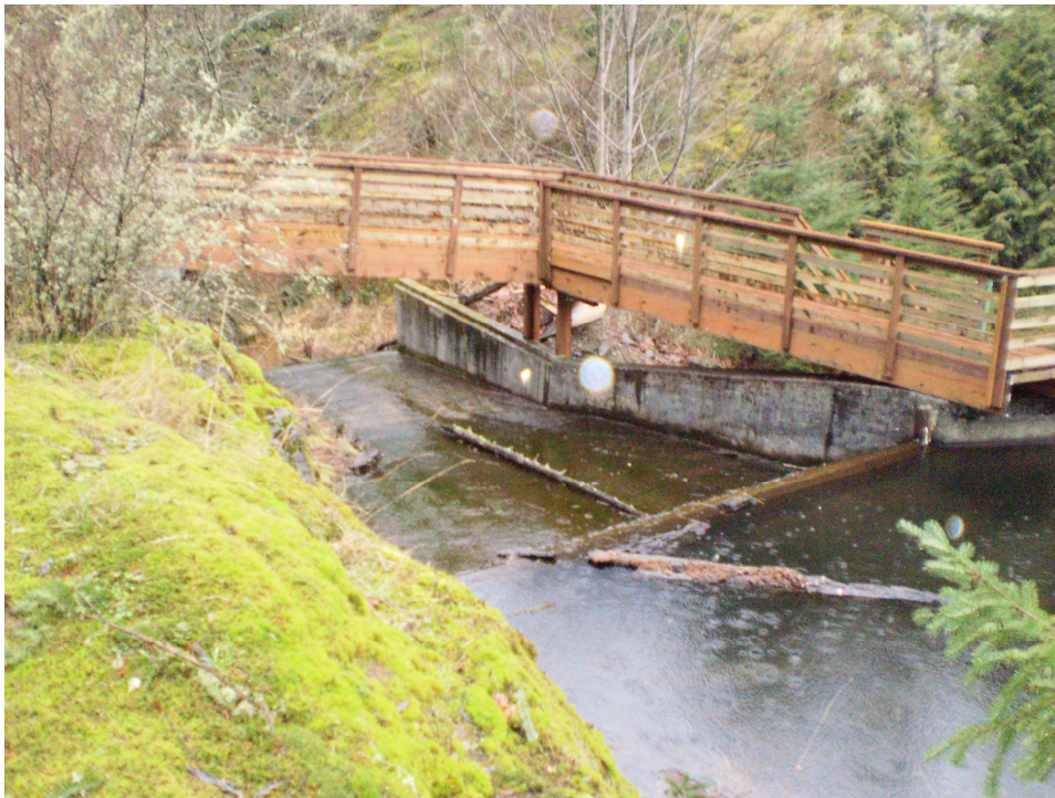
Photo No. 2 View spillway from left abutment
