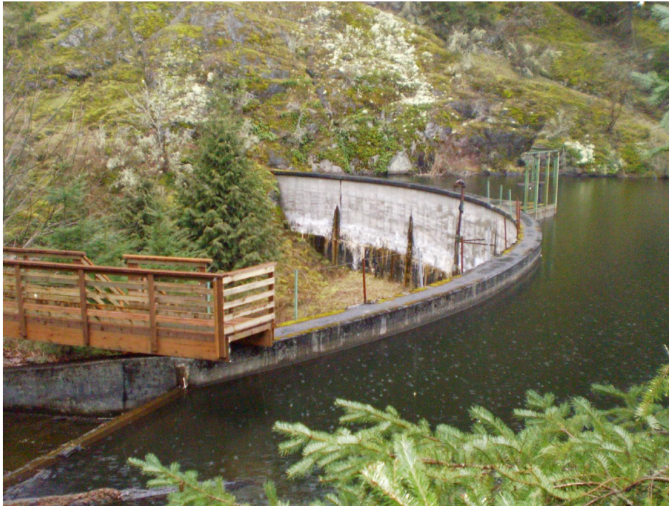
Photo No. 1 View dam from left abutment
