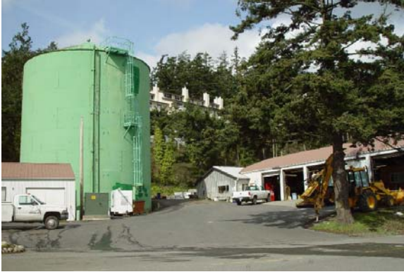
Water tank and Public Works Department
